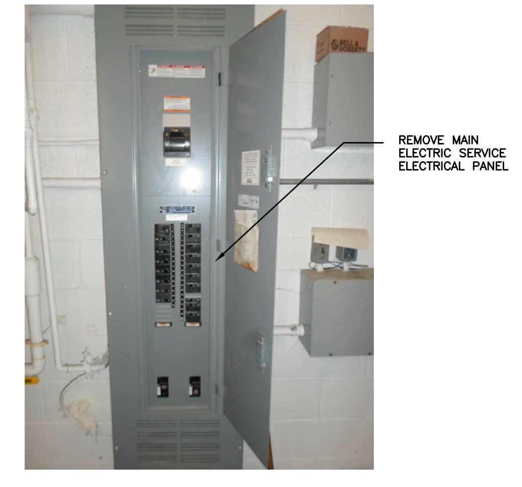
3 MAIN SERVICE ELECTRICAL PANEL NTS
