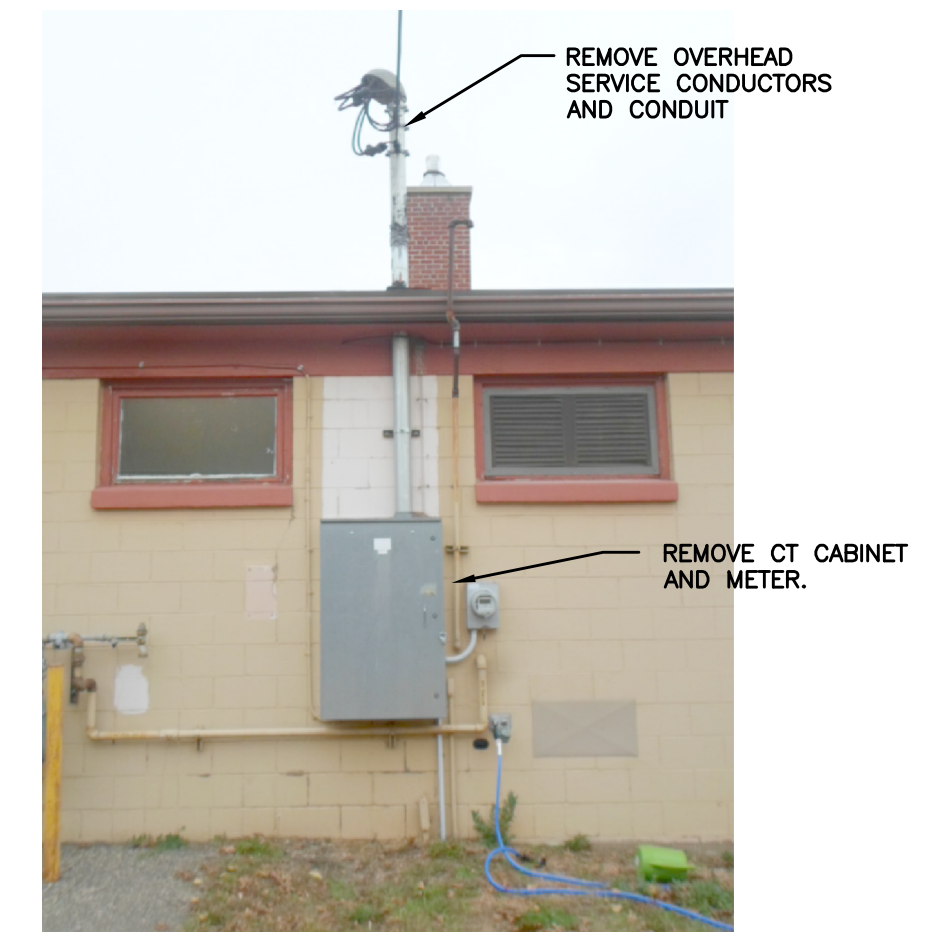
2 CURRENT TRANSFORMER CABINET NTS
